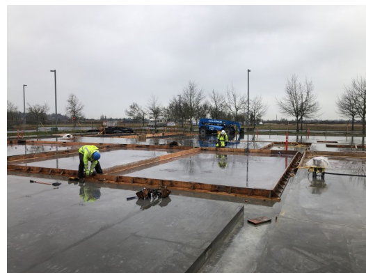
Pouring Panels at Market of Choice
