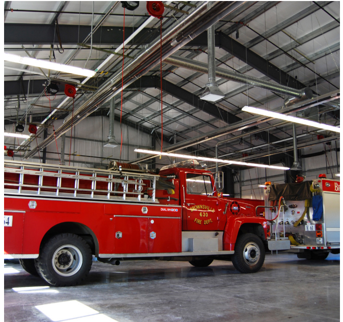
Station #61 - Pre-Engineered Metal Apparatus Bay
